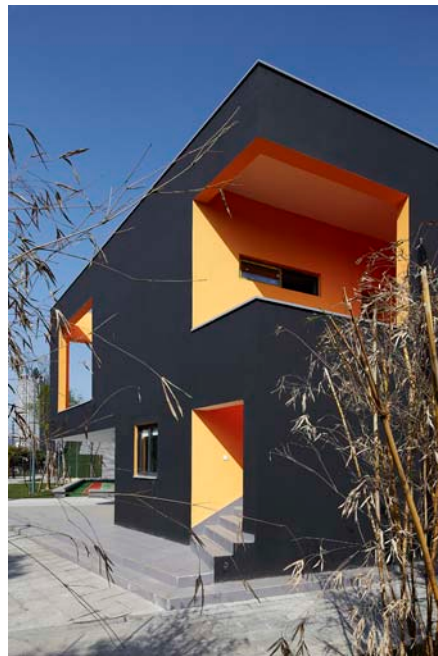
三瓦窑附属用房 (Annex House of Sanwayao)
