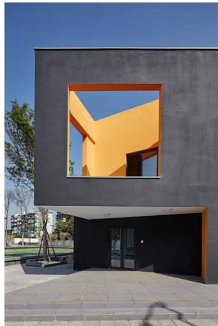
三瓦窑附属用房 (Annex House of Sanwayao)
