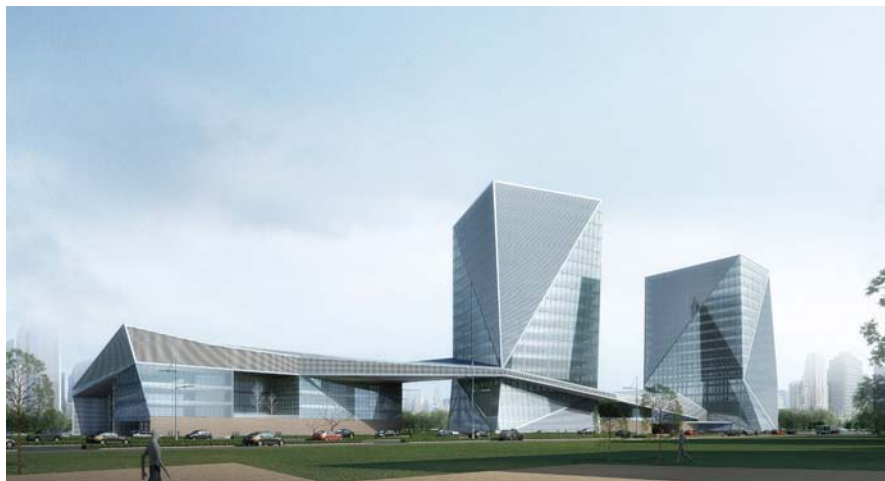
公安局办公楼 (Office building of public security bureau)
