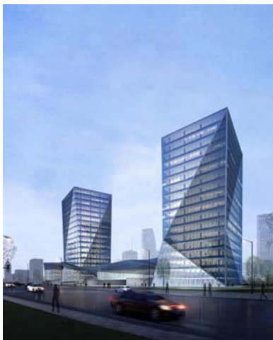
公安局办公楼 (Office building of public security bureau)
