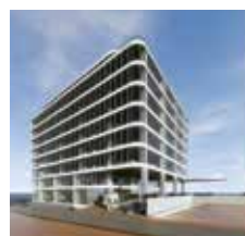
YANGON OFFICE TOWER
