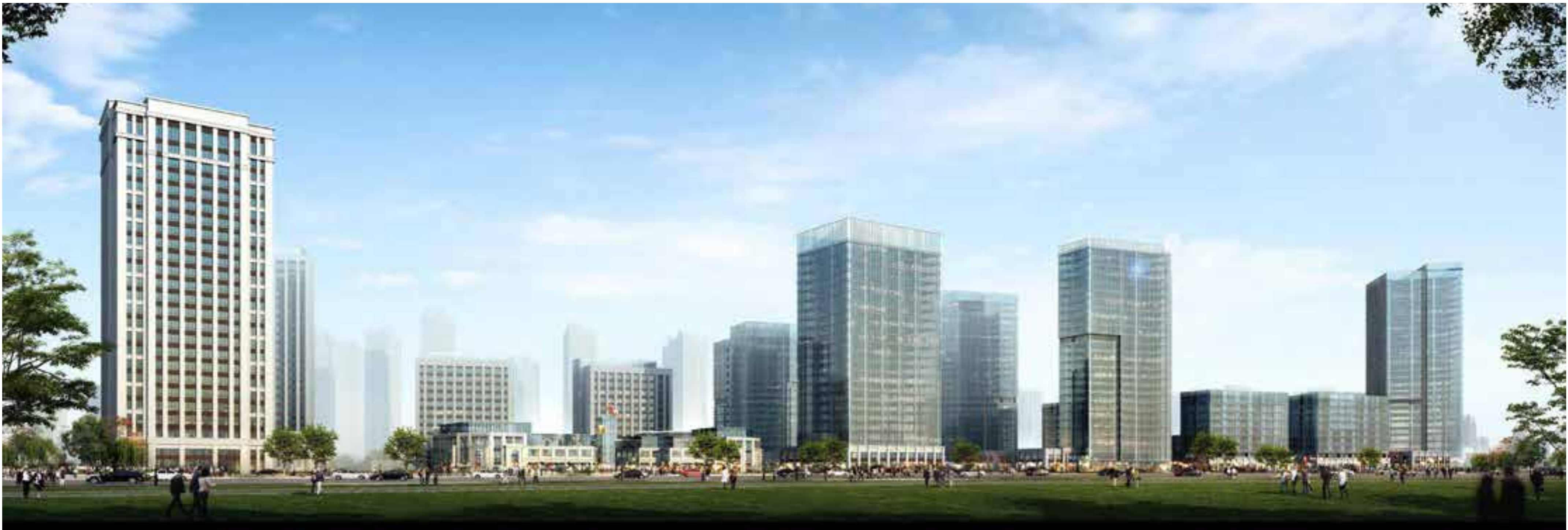
The Commercial Building 1、2 & 3 Of R&F New City In Xianghe
