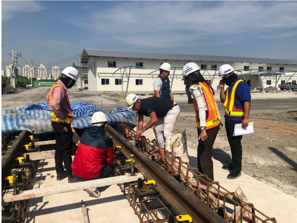
Figure9 Controlling installation of Mockup Track Plinth
