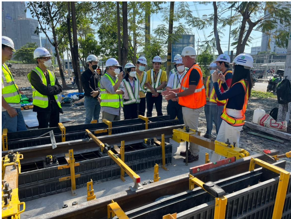
Figure10 Controlling installation of Mockup Track Plinth
