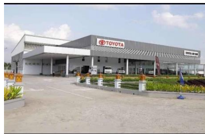
Toyota Car Showroom Project
