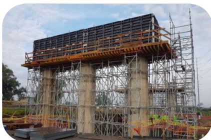
Shoring structure design work
