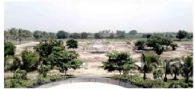
Memorial for Smt. Shilaben Modi (under construction)
