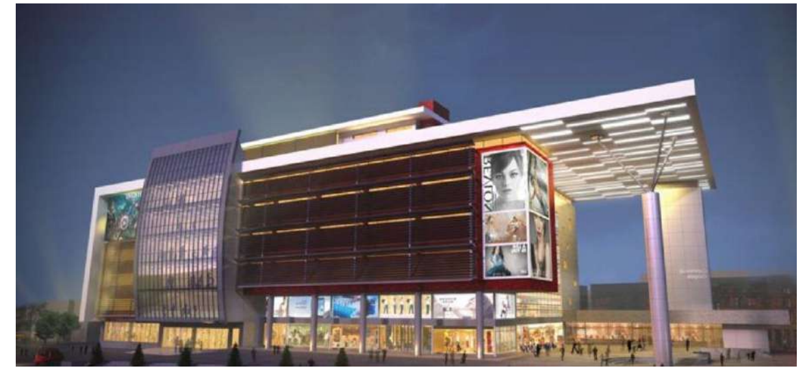
VIEW FROM MAIN ROAD
