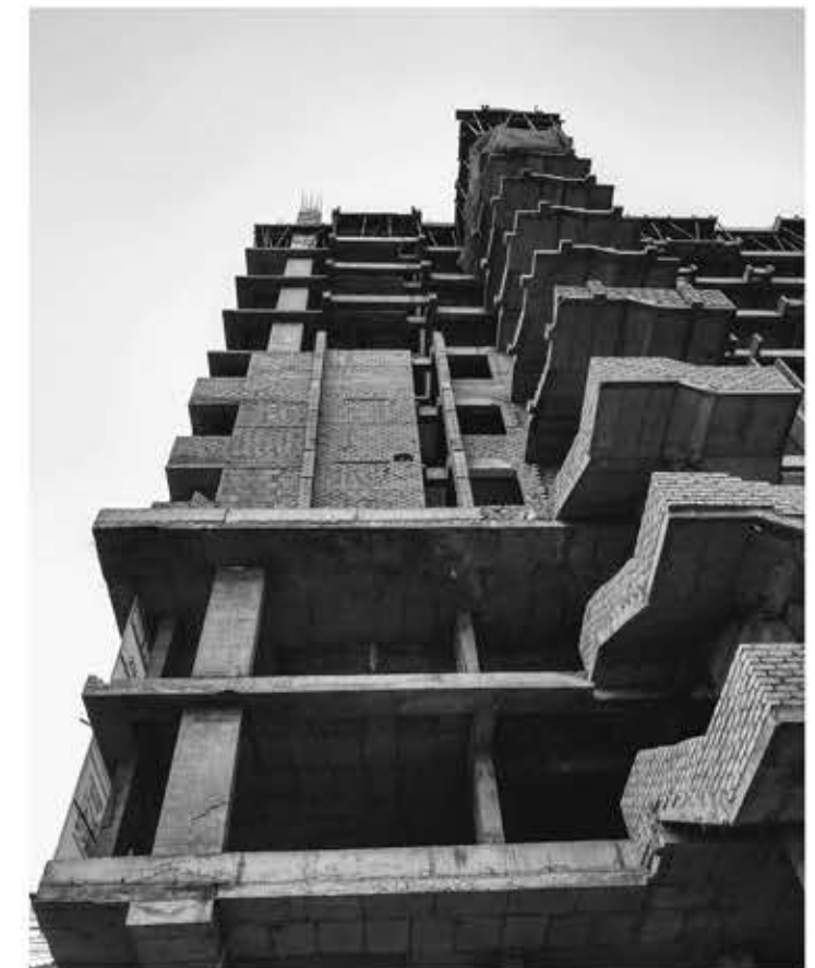
Under construction site, Jaipur
