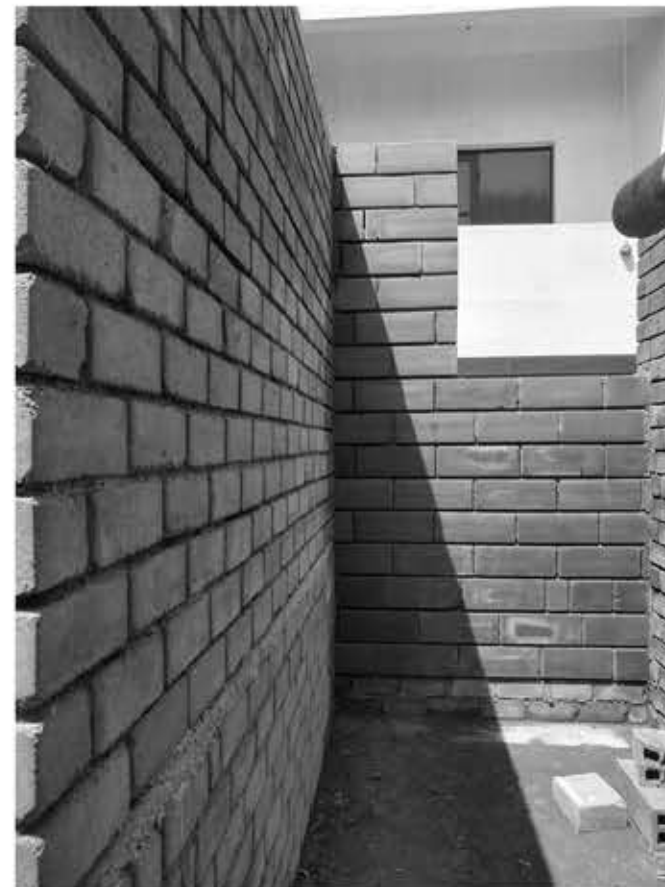
Under construction site, Jaipur
