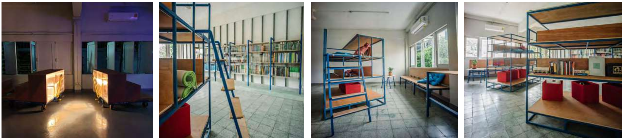
Location: Entrance at Nakornsawan Road, 77 Entrance, Wat Sommanat, Pom Prap Sattru Phai, Bangkok 10100 Date: August 2019 - October 2019 Role: Architect Assistant, Onsite Worker By: Space Saloon Studio Sponsor: Ford Resource and Engagement Center(FREC Bangkok)
