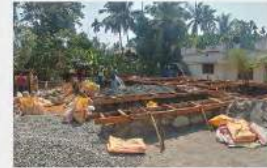
Plinth beam shuttering
