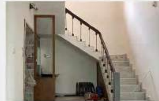
interior site work
