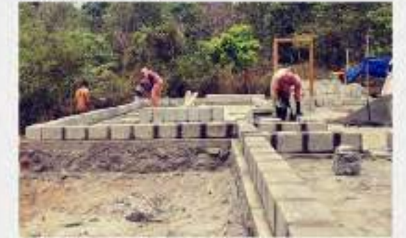
Ground floor masonry works.
