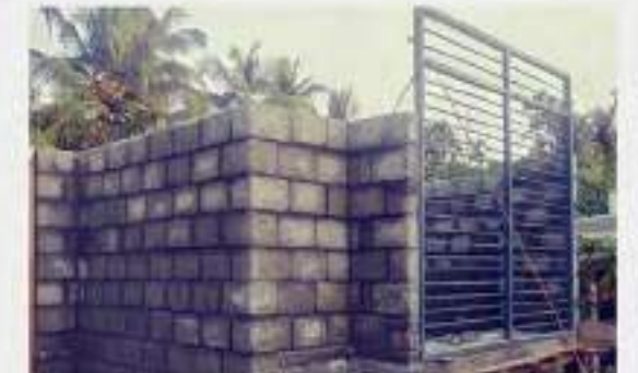
bay-window designed being installed and masonry works reaches lintel level.
