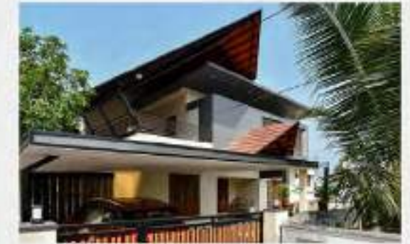
Front view after
