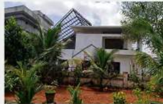
exterior truss work
