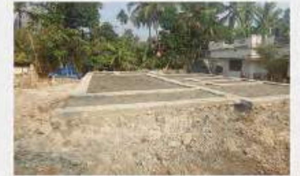
Plinth beam setting
