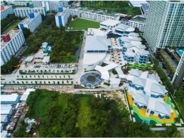
Shrewsbury international school 4 buildings
