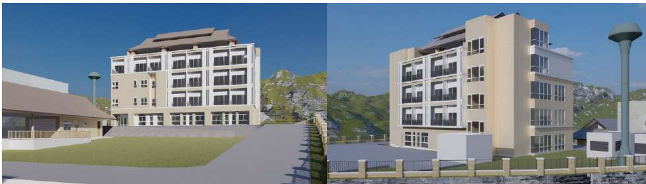
IPD & STAFF BUILDING
