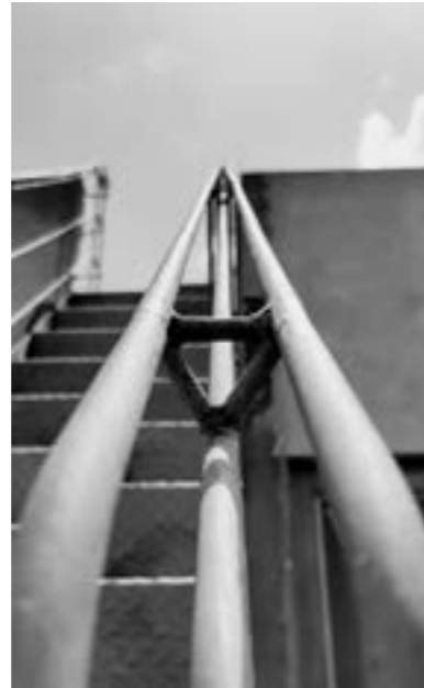
Triangulated grab bar Three MS rods combine with intermediate ties to form a steady grab bar
