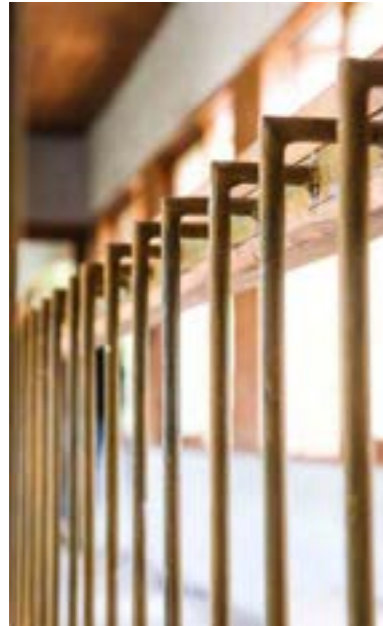
Wood - metal union kinked MS handrail welded to MS plate fixed on 2'x 2'teak wood
