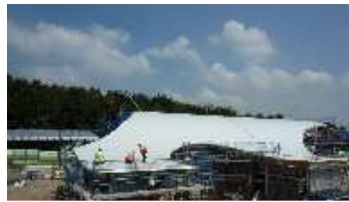
roof : smart board with Evalon waterproof membrane
