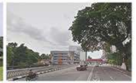
4 Jalan Sultan Idris Shah Birch Bridge
