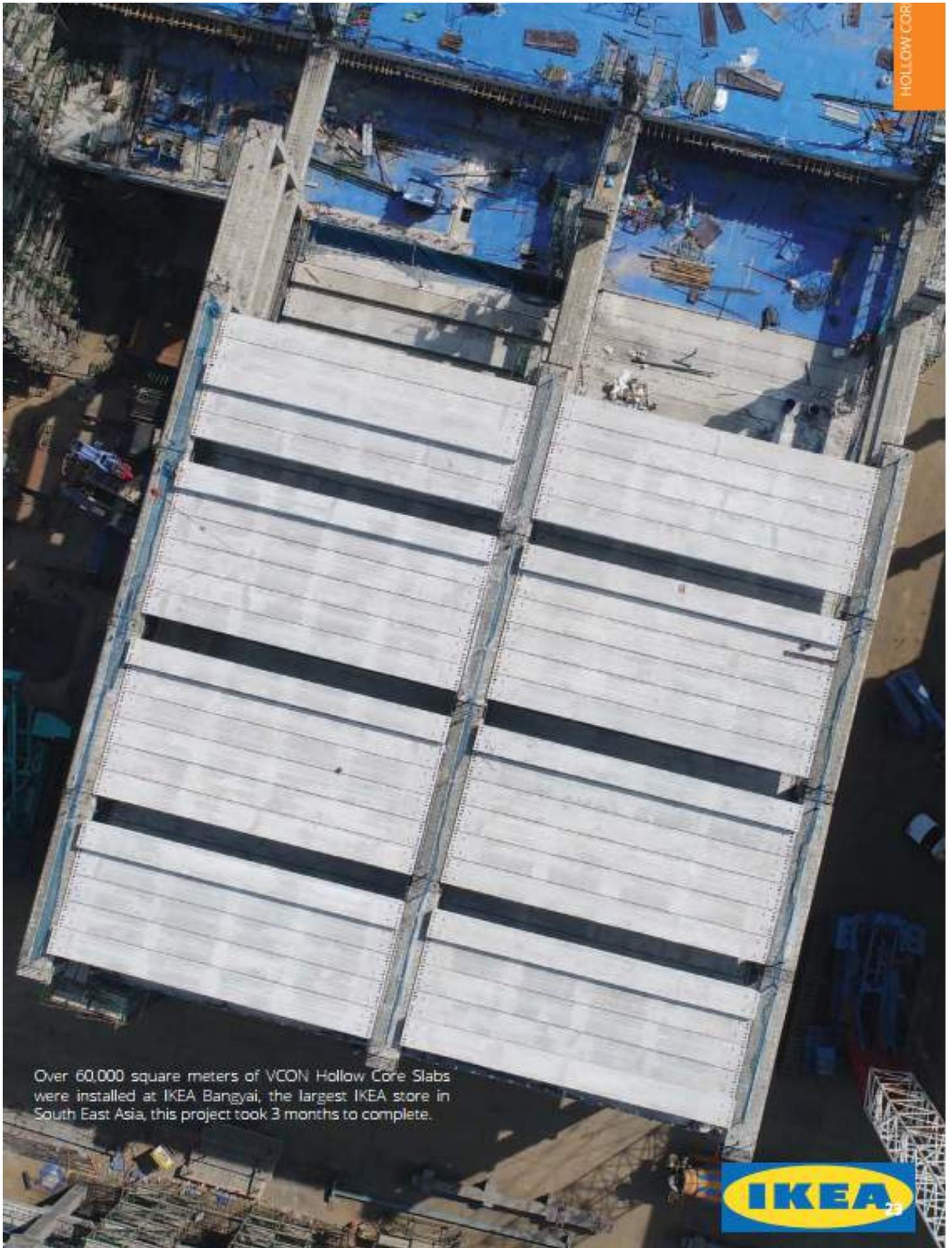
Over 60,000 square meters of VCON Hollow Core Slabs were installed at IKEA Bangyai, the largest IKEA store in South East Asia, this project took 3 months to complete.
