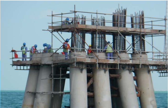
Design of Temporary Bracing for Breasting Dolphin Piles
