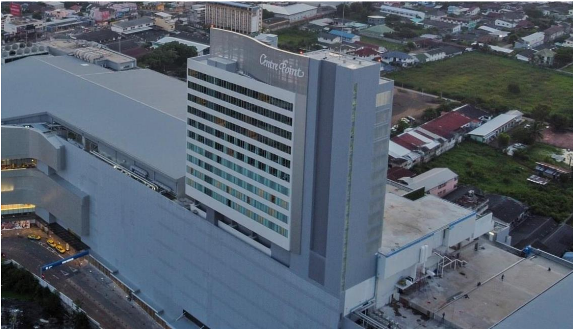
Pic 4 18 th Floor for Retail & Hotel Building , Total Height 92.65 m.
