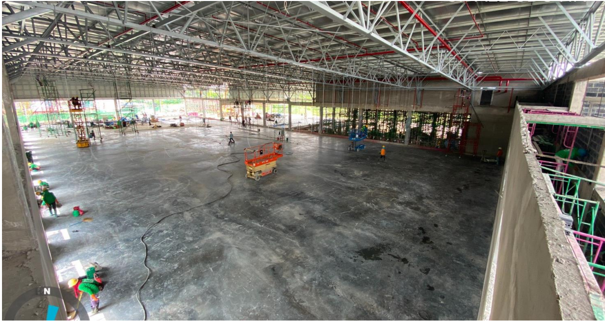
Pic 3 Steel Truss 30 m. long span for metal sheet roof.
