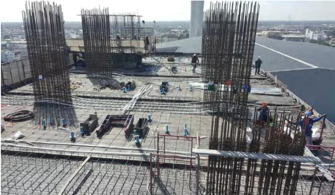
Pic 3 Post-Tensioned slab for typical floor
