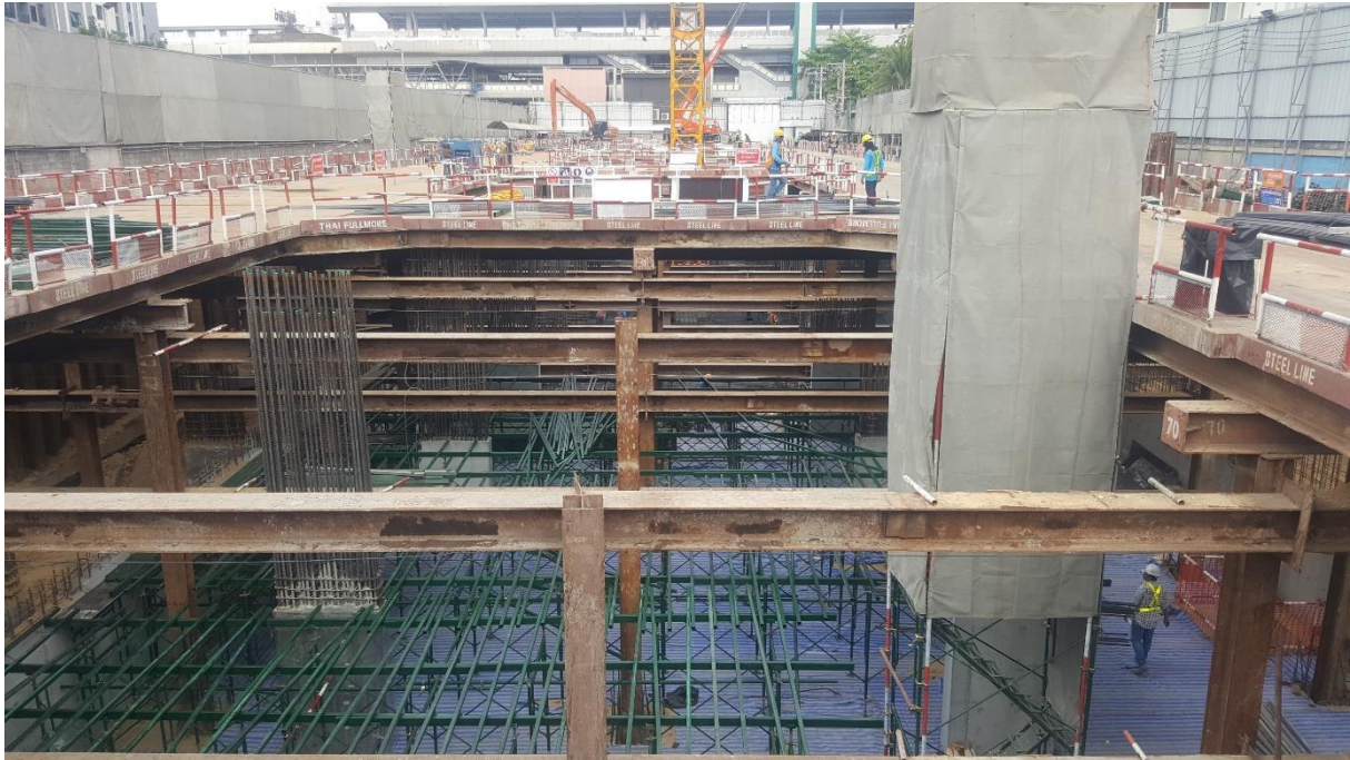
Pic 1 Sheet pile with strutting system for construction 2 nd Basement floor.
