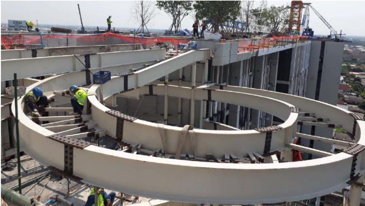
Pic 3 Spiral Steel Bridge Link between tower on 15 th Floor.
