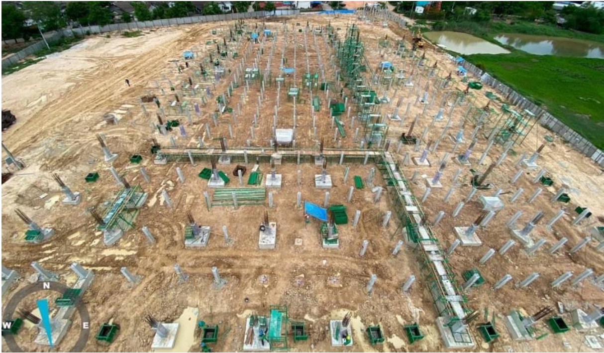
Pic 1 PC. Driven Square Pile for factory and warehouse building.
