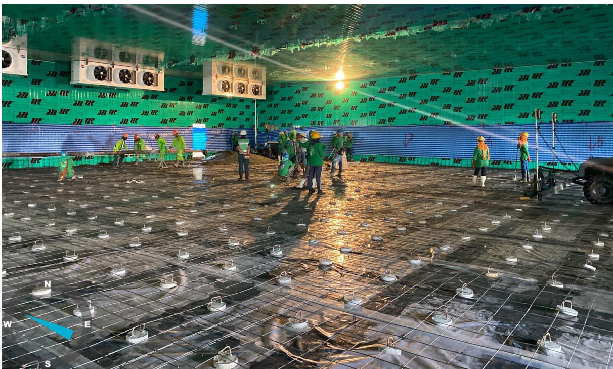
Pic 4 RC. Flat Slab with Topping for freezing zone.
