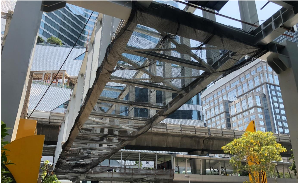
Pic 3 Steel Vierendeel Truss for 30 m. long span bridge above Ploenchit Road.
