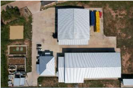
Asano Ginger New Factory @Payao (110 M Baht) Completed on 2022
