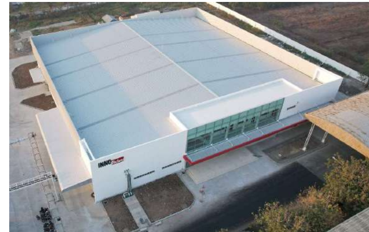
INNOValue New Factory @Ayutthaya (100 M Baht) Completed on 2023
