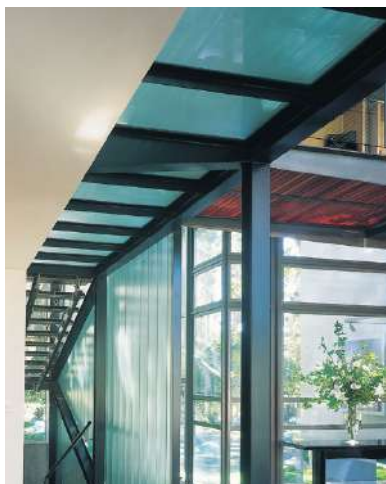
Figure 1-8: 440 House, Palo Alto, California, USA, 2000; Tapered beam application in a modern resident
