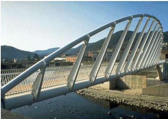
Figure 1-4: La Devesa Bridge, Ripoll, Spain, 1991; Tapered arms that serve to transmit load from deck to arch
