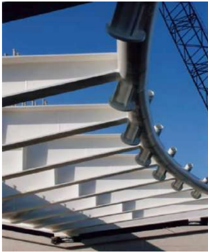
Figure 1-3: Three Bridges over Hoofdvaart, Amsterdam, 2004; Tapered beam along the bridge length
