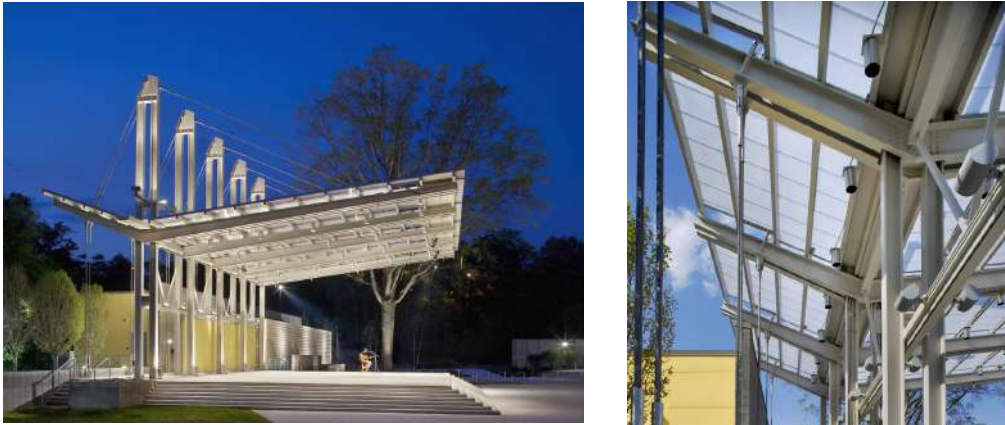
Figure 1-6: Fayetteville Festival Park, North Carolina, USA, 2004; the canopy was fabricated from tapered wide flanged steel sections
