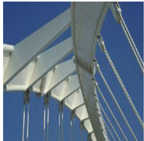
Figure 1-4: La Devesa Bridge, Ripoll, Spain, 1991; Tapered arms that serve to transmit load from deck to arch
