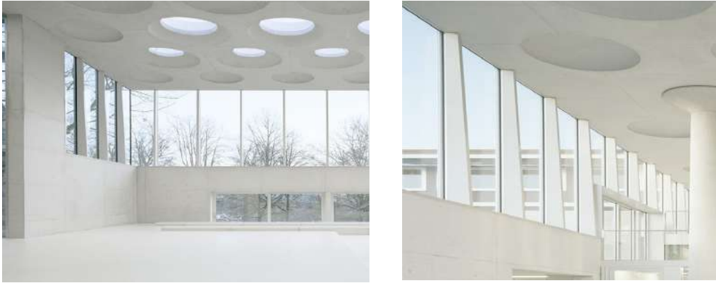
Figure 1-9: Forum at the Eckenberg Academy, Adelsheim, Germany 2013; tapered steel columns integral to the curtain wall façade transfer the remainder of the roof loads
