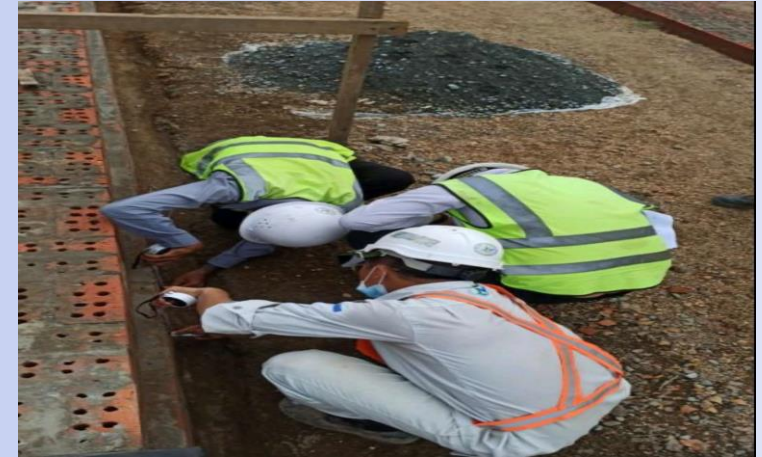
Inspection the completed work activities with consultant parties
