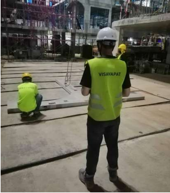
Installation of Precast work
