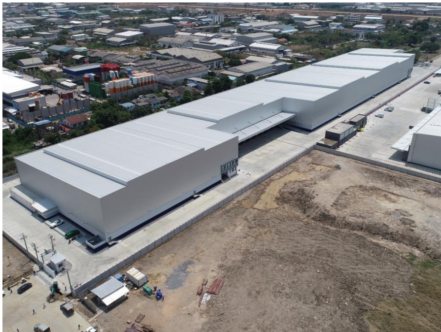
FIG.6 Bird eye view at Yellow Wood 6 New Warehouse
