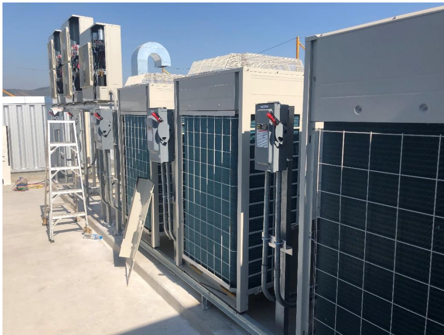
FIG.14 CDU area (Roof slab) at ASRB New Factory
