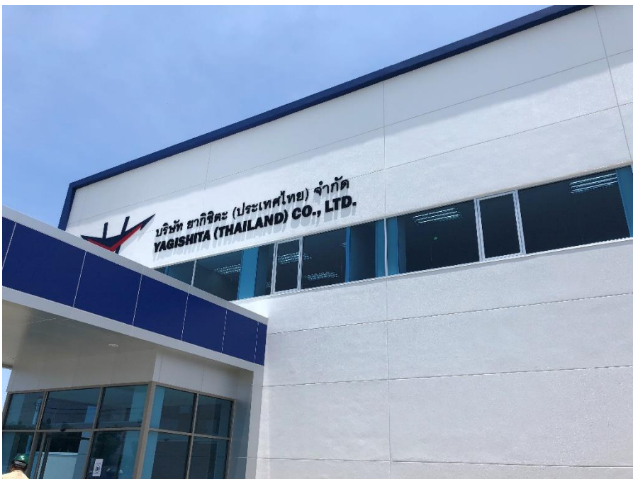
FIG.4 External area (Front) at Yagishita New Factory
